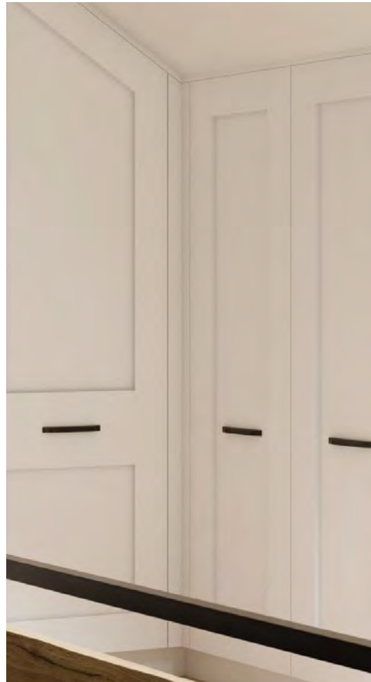
Plinth used to create corner post
