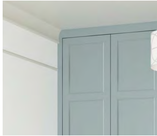
Plinth used as infill to ceiling
